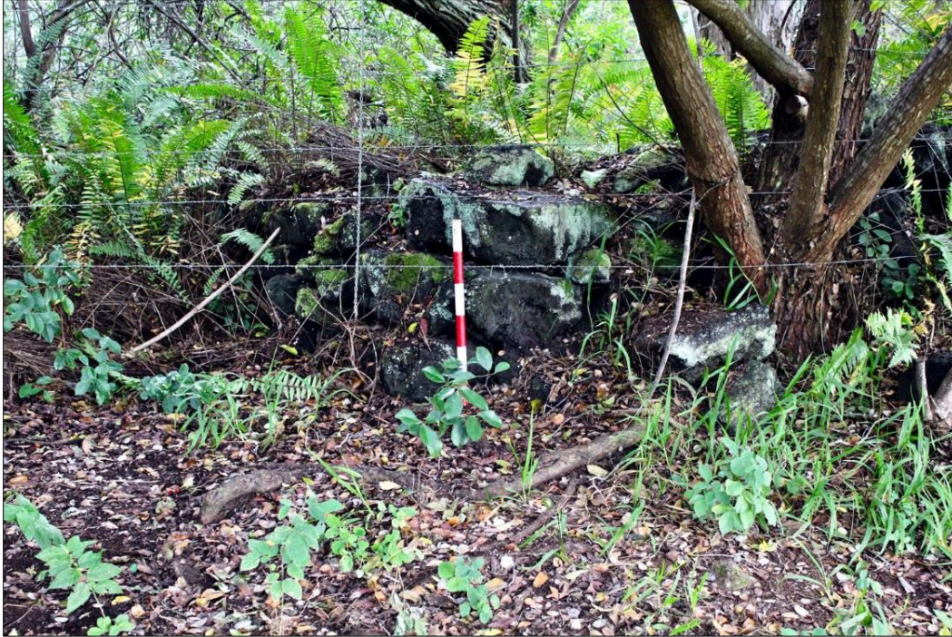
Figure 26. Southeastern corner of the wall surrounding Haunakalili pit, view to the northeast.
